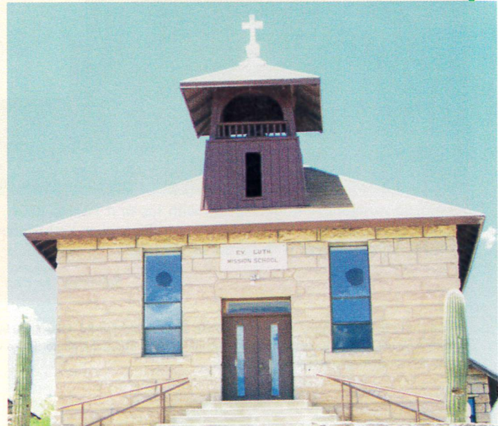
Peridot Lutheran Church after it was vandalized.
