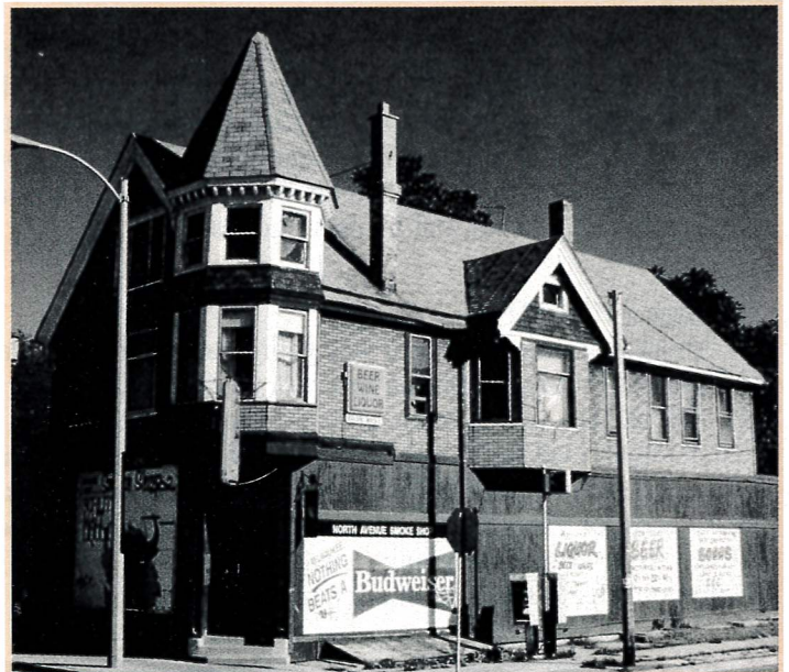
An old smoke shop and liquor store is the site of a new ministry center in Milwaukee. The ministry will reach out to the community from this building, which was purchased for $1 and renovated by Builders For Christ.
