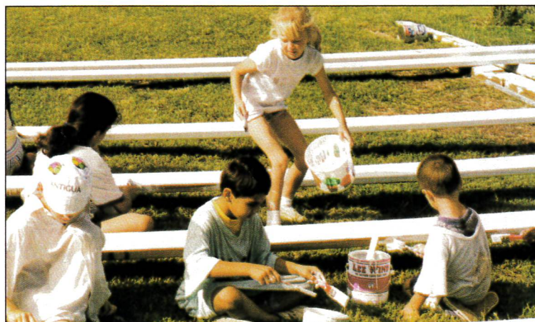
No one is too young to help. St. John school children helped paint the boards used to repair the school's gallery roof.
