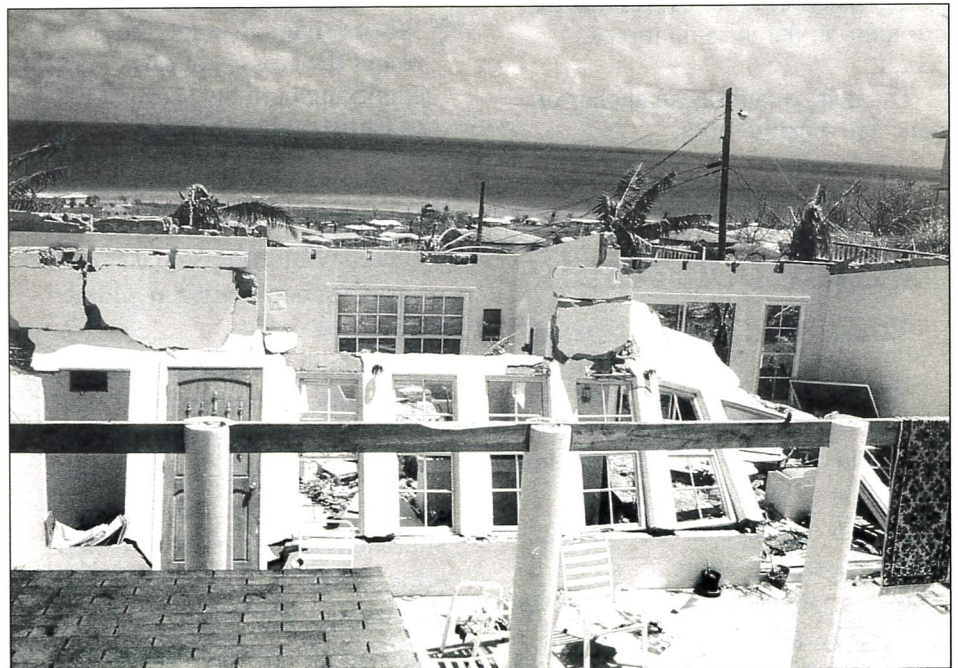
The Kehl home was destroyed by Hurricane Luis. The house weathered the storm for 12 hours until the wind shifted and caved in the entire front wall.
