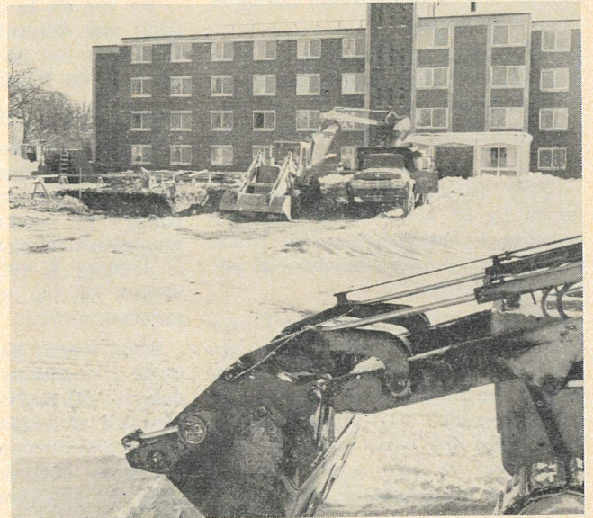
Heavy Equipment at work
