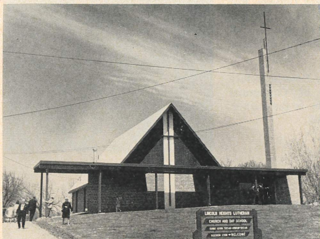
LINCOLN HEIGHTS LUTHERAN, Des Moines, Iowa, presents this view to one coming up the hill.
