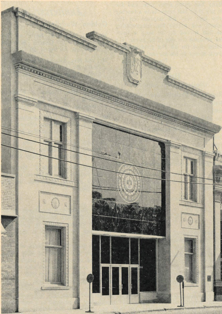
AFTER remodeling. This is now the Administration Building of the Wisconsin Evangelical Lutheran Synod. The seal of the Synod is in gold on a field of black marble.
