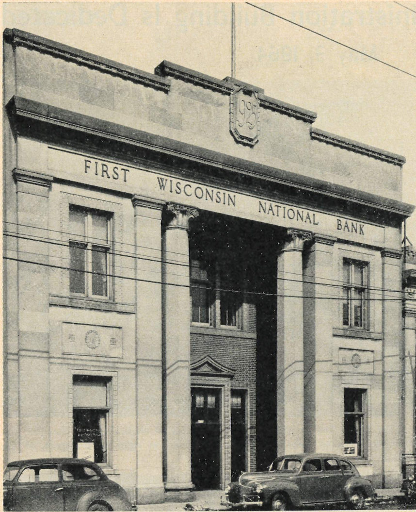
BEFORE remodeling. The building was used for banking purposes from 1925 to 1960. This picture was taken in 1946.
