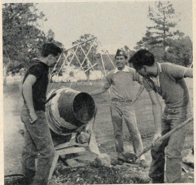
The Boarding School boys help with the construction work at the Mission
