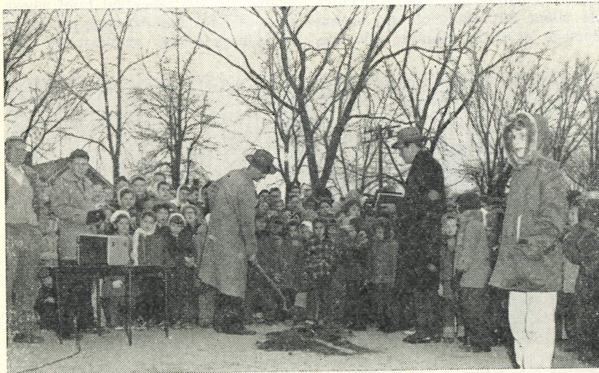
Breaking ground for new addition to Friedens Lutheran School, Kenosha, Wisconsin
