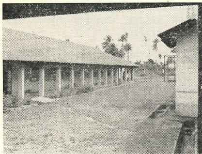
The women's ward at the Lutheran Hospital at Eket
