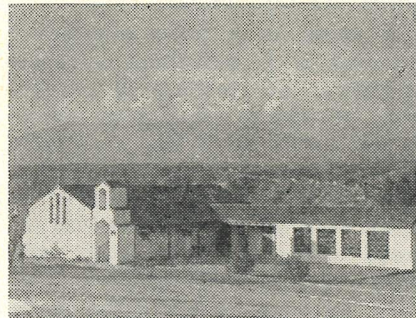
St. Peter's Ev. Lutheran Church and New Sunday School Wing Just Nearing Completion
