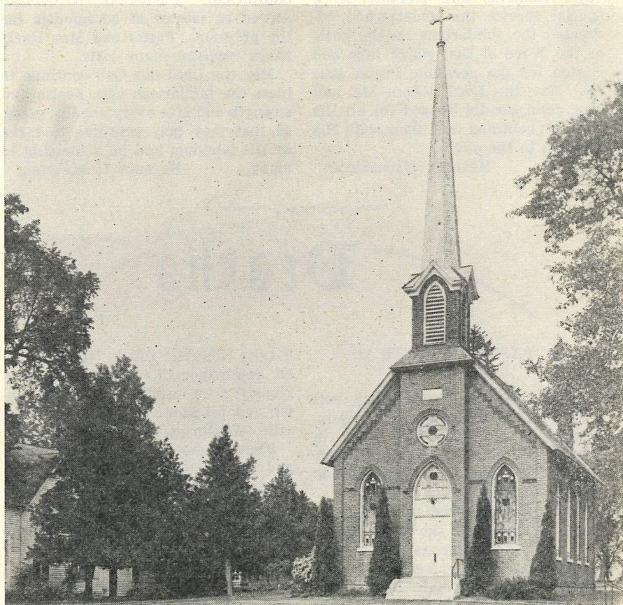
St. John's Ev. Lutheran Church, Baytown, Stillwater, Minnesota
