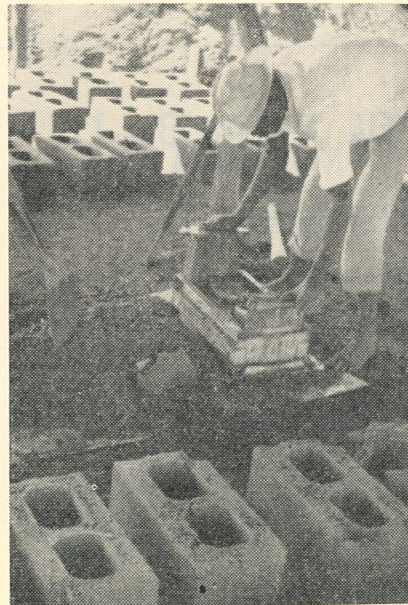
One of our native workers making our cement blocks. Two of our workers pleaded for advance in salary so they could get wives. One asked for $15.00, the other for $12.00.
