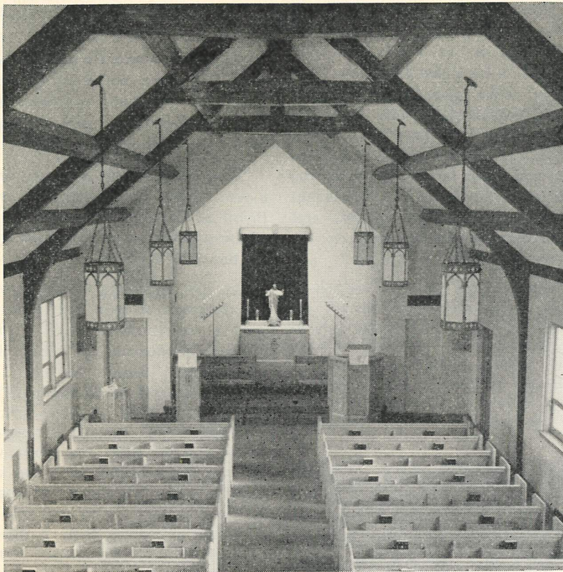
INTERIOR, CHRIST EV. LUTHERAN CHURCH
