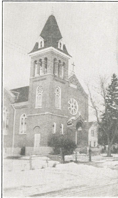
St. Paul's Evangelical Lutheran Church, Town of Franklin, Milwaukee County
