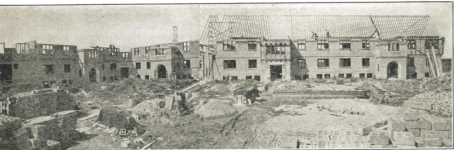
a view of the building site taken on August 29th
