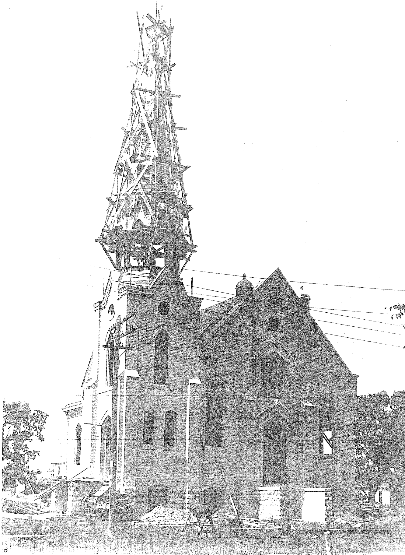
St. Paul's Evangelical Lutheran Church under construction in 1909.
