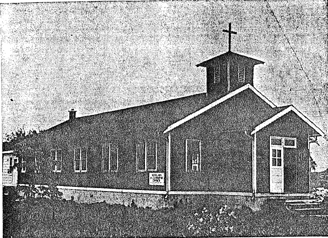
REVIVED—An old church building that served the St. Matthew's Lutheran congregation at Oconomowoc for many years, and then was discarded with construction of a new building, is seeing use once again in Milwaukee. Cut into sections, the church was moved to Milwaukee to be reconstructed and is now serving as the gathering point for the newly organized Westlawn Lutheran congregation in that city. (Freeman staff photo)
